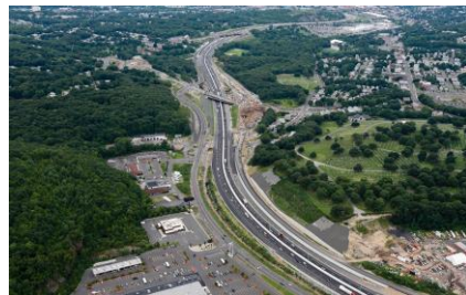
I-84 Waterbury Improvement Program
